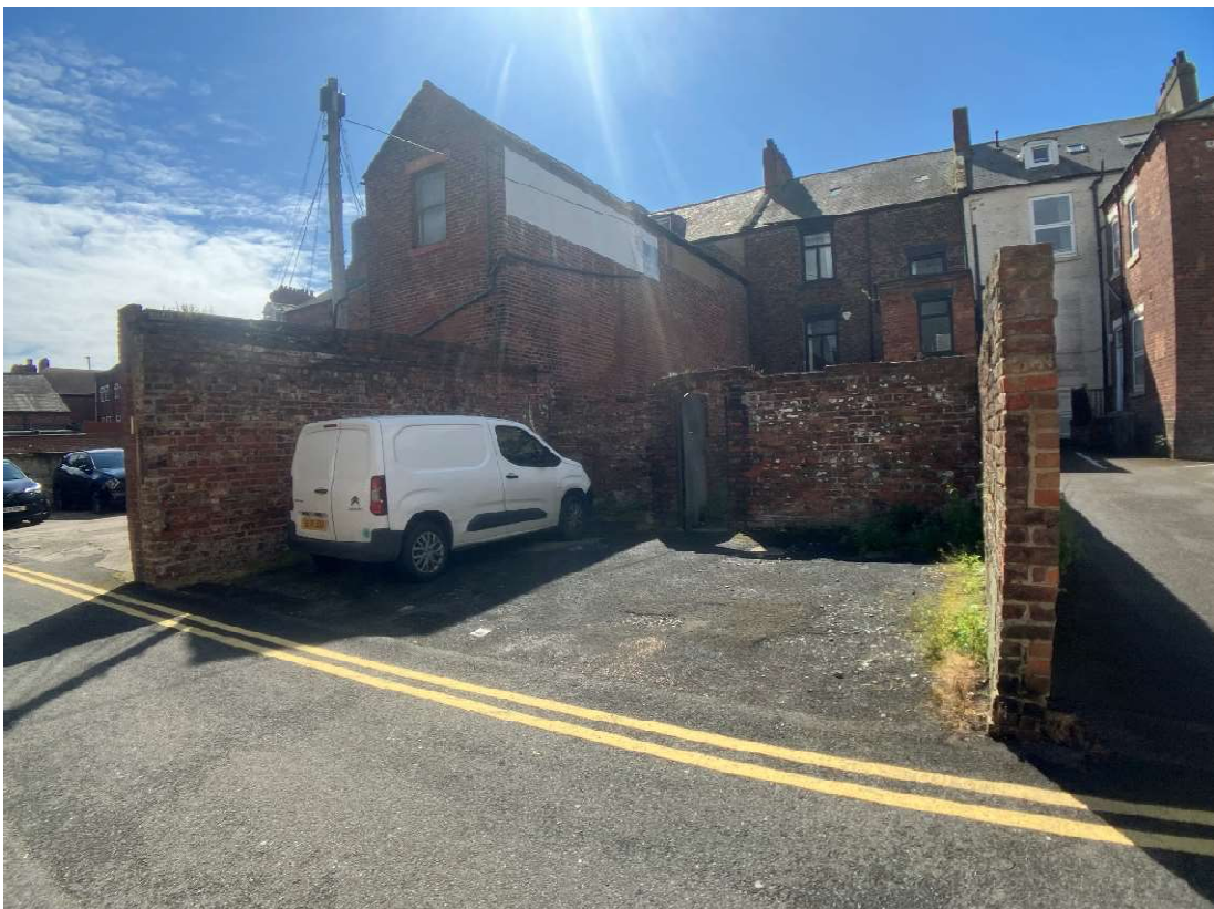
View from unadopted road of rear façade
