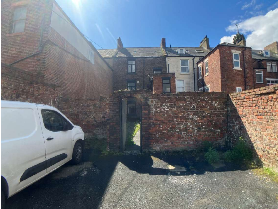
Rear Façade from car parking area
